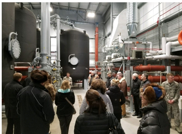
Eielson AFB Water Treatment Plant Granular Activated Carbon system.
