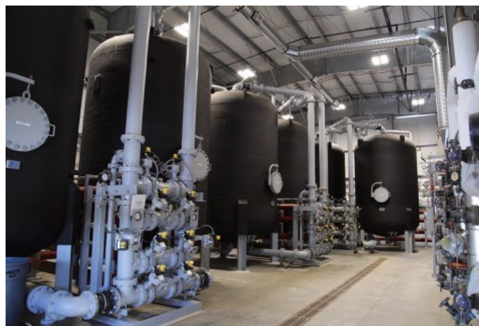
Eielson AFB Water Treatment Plant Granular Activated Carbon system.
